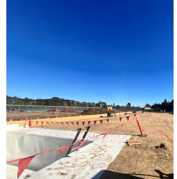
12/11/2025 South Building Elevator Pit
