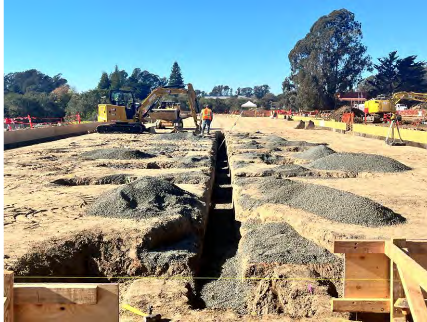
12/11/2025 South Building Underslab Plumbing
