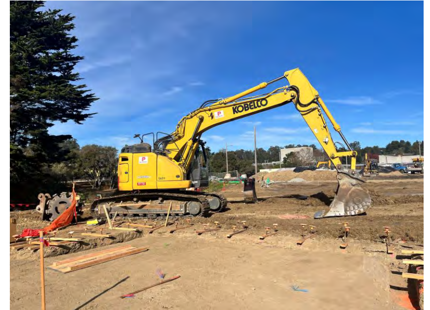
12/18/2025 North Building Edge Form in Progress
