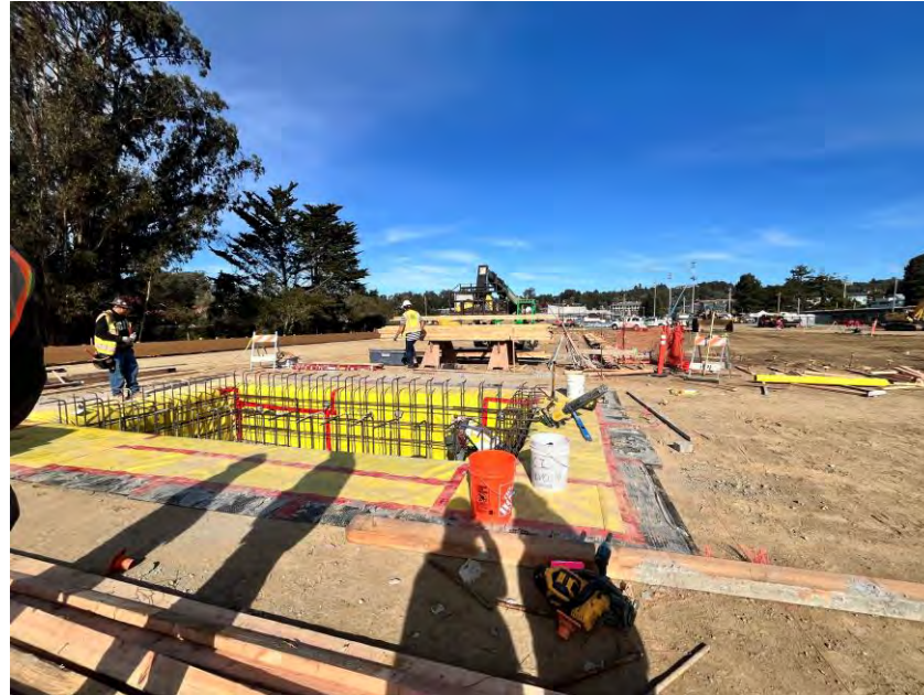
12/18/2025 Central Building Elevator Pit Prepped for Concrete Casing
