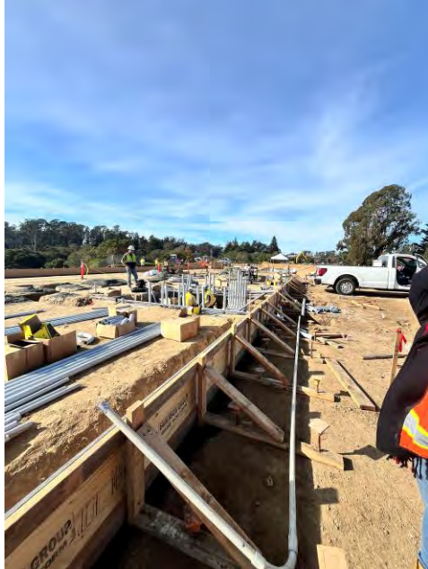
12/18/2025 South Building Underslab Plumbing and MPOE
